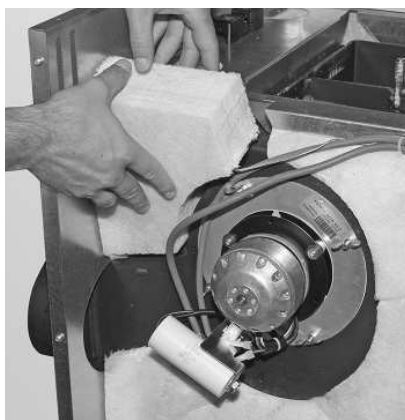
Fig. 34 Attach the insulation (included, on side at base of induced draught fan)
