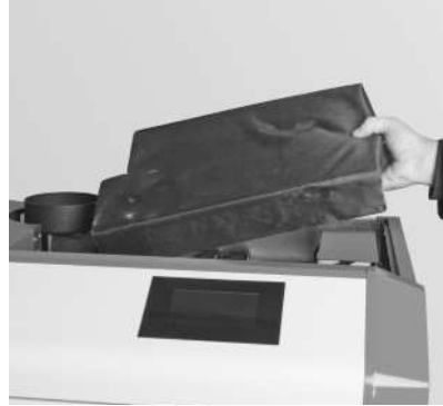
Fig. 97 Apply insulation
