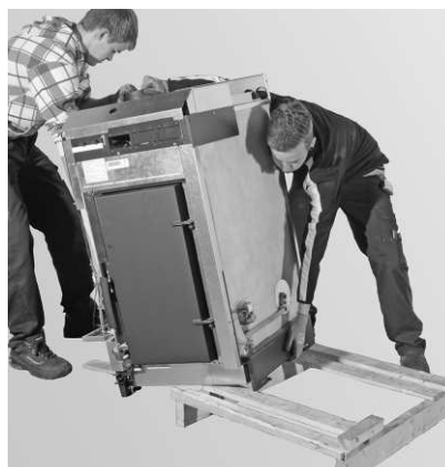
Fig. 10 Move boiler off pallet
