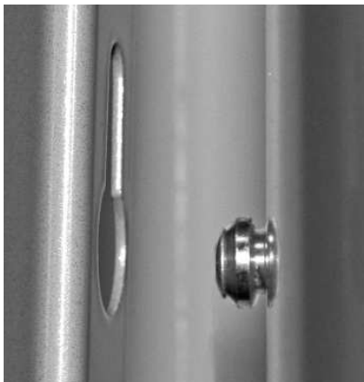
Fig. 72 Bayonet lock
