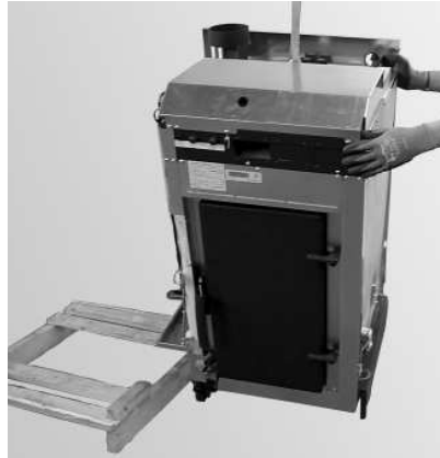
Fig. 14 Lift the boiler off the pallet
