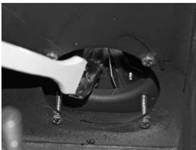
Fig. 56 Clean and vacuum the induced draught fan wheel
