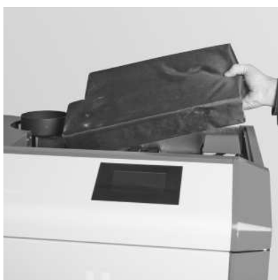
Fig. 63 Remove the insulation
