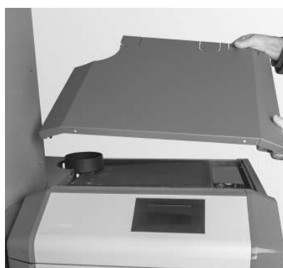
Fig. 62 Lift off the top cover
