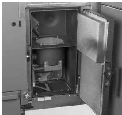
Fig. 4 Open the combustion chamber door during the filling process
