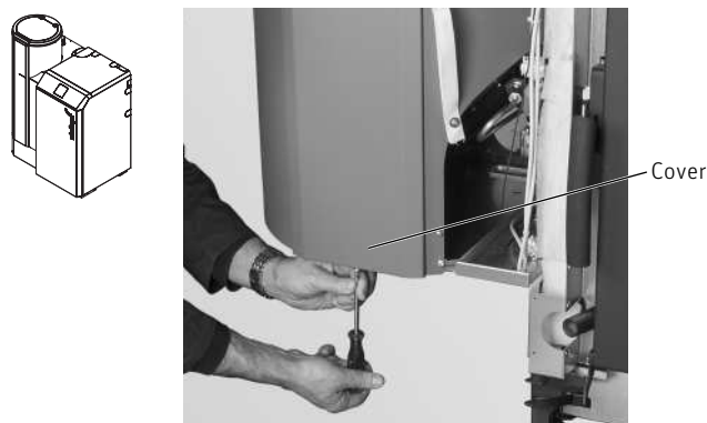
Fig. 45 Dismount the cover, removing 1 screw
